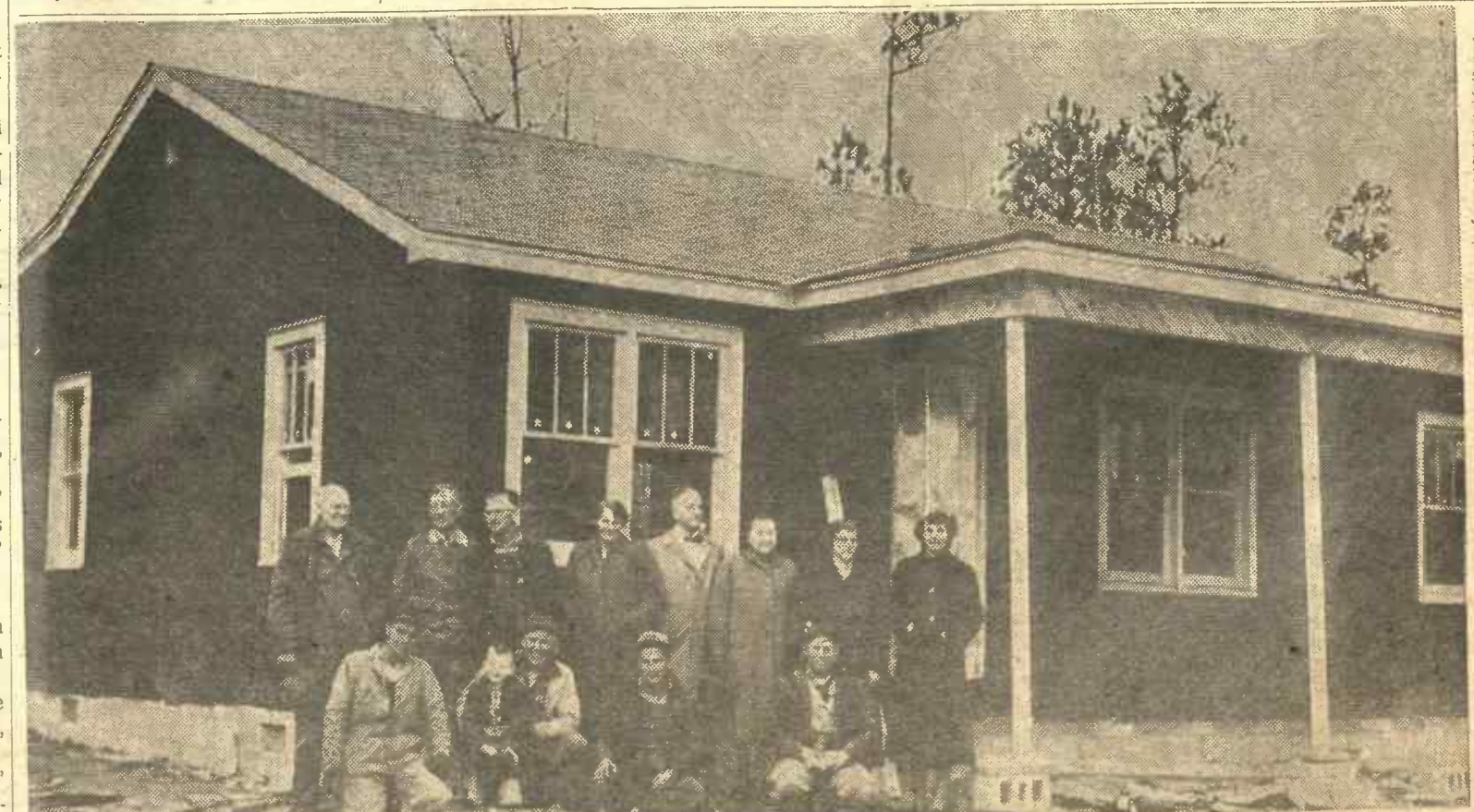
UNDER CONSTRUCTION — THE new pastor's home for the New Prospect Baptist church is pictured above during its construction. The New Prospect community is four miles south of Iuka and the church and pastor's home are located just off highway 25. The church has 150 members. Construction of the parsonage is being done principally by volunteer labor. It is a nice six-room bungalow and will have all modern conveniences. Shown in the picture are
